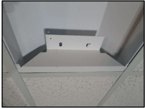
PICTURE OF ENDCAP INSTALL SEE FIG 02
