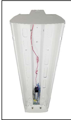
STEP 3 REMOVE BALLAST COVERS
