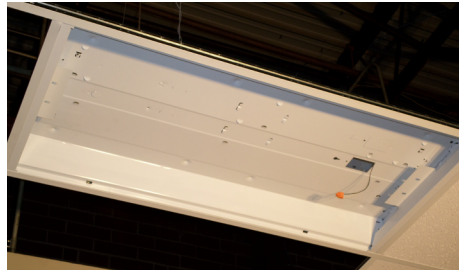
2) Insert endcaps between ceiling grid and troffer.
